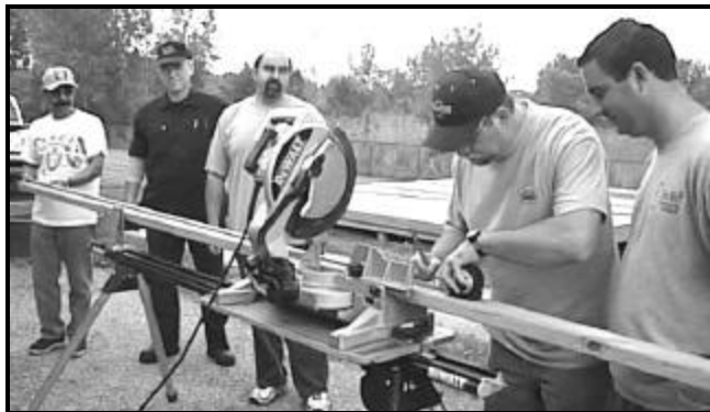
From left Juan Guajardo, Ron Gluth, Sam Rodriguez, Merrill Clark and instructor Shawn Myers, measure and cut handrails for the LCAR deck.
